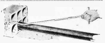
A socket wrench with a universal joint to reach normally inaccessible points has been produced by the Bell Telephone Laboratories of New York City.
